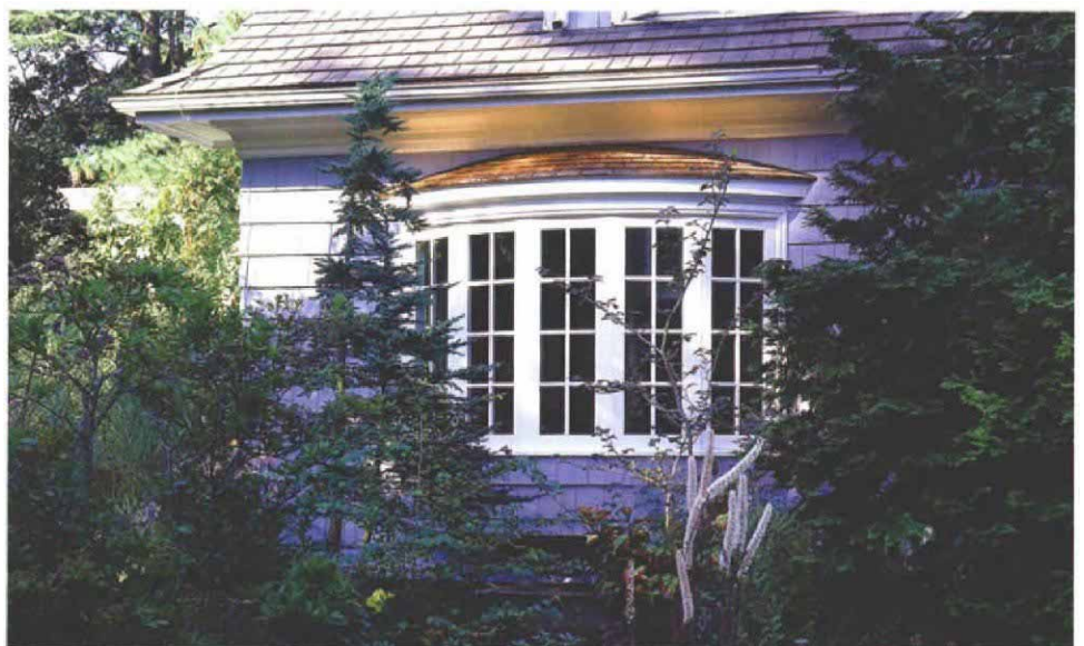
Custom curves. A bow window built by the author looks right at home on this Seattle bungalow-style house (above) while offering great views of carefully tended gardens from the inside (top). Window sash is flat, but trim pieces are laminated curves.
